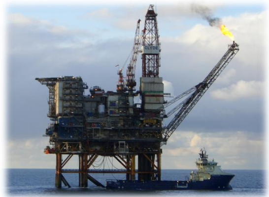
Figure 1 : Rig and Support Vessel
