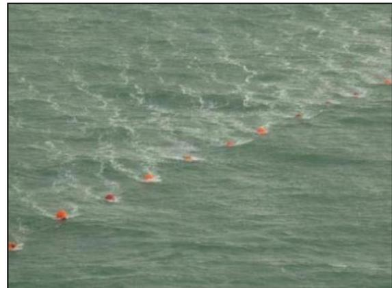
**Figure G:** Floats left on cable for 24hrs landing
