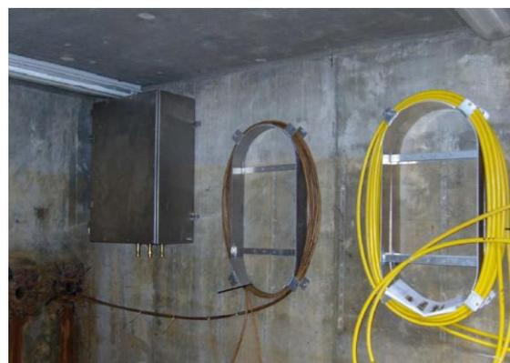
**Figure 6:** Power Switch in Beach Manhole
