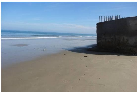
**Figure 5: Vertical seawall reflects wave energy but does not dissipate, exacerbating erosion**
