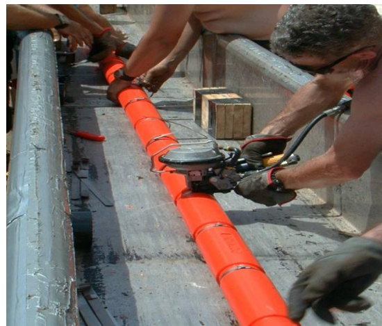
Figure 4: Polyurethane covering for 30mm separation between cable and pipeline.
