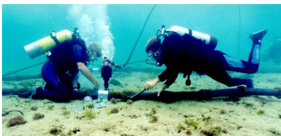
Figure 5: Attaching Articulated Pipe
