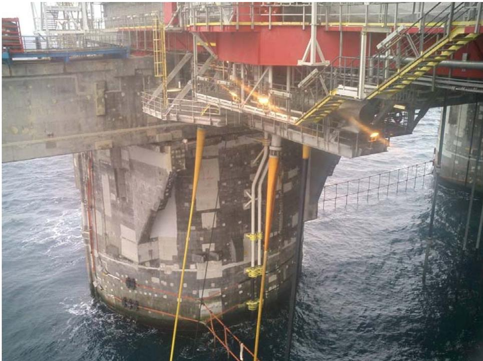
Fig 1 Dynamic riser cables installed at a platform
