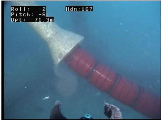
**Figure 4: ROV Monitoring and Inspection of Bell-mouth**
