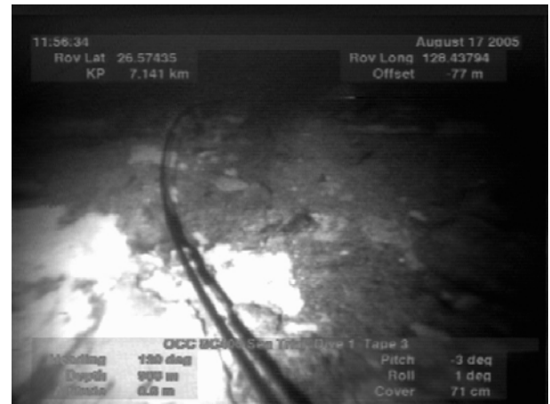
Figure 7: The meanderer of laid cable
