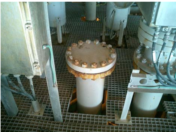
Figure 3: Riser top flange
